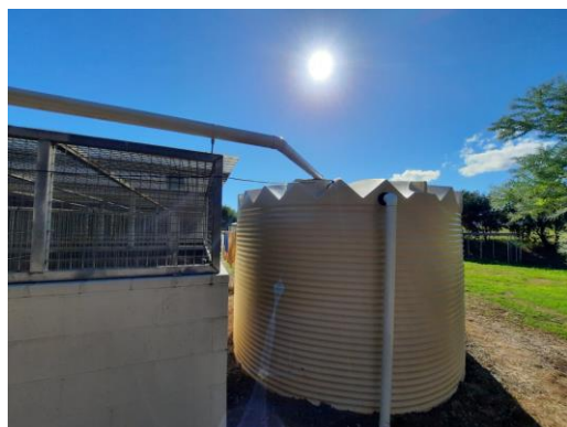
Figure 4 and 5: Rainwater tank and spray system installed at the Tamworth Pound
